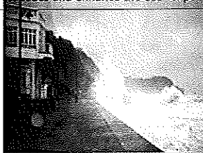
Overtopping is when water passes over the top of the sea defence crest line.
